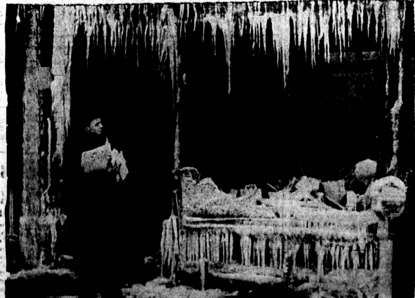
Wondering where to deliver his mail, postman Robert Freeman is seen surveying icy remains of one of two stores which was gutted, along with Masonic hall, by $500-
