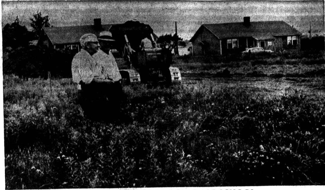
BREAK GROUND FOR NEW PARKDALE SCHOOL
