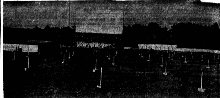
The newly named "North River" Drive-in Theatre at West Royalty is attracting much interest as the opening date draws near. The huge screen contains 114 sheets of three-quarter inch plywood, painted white. A plywood fence will shield the field from the glare of car headlights. The portion of fence near the screen is eight feet high while that farther away is four feet. The canteen building, shown at the left, is built of concrete blocks.—(Photo by Margaret Mallett).
