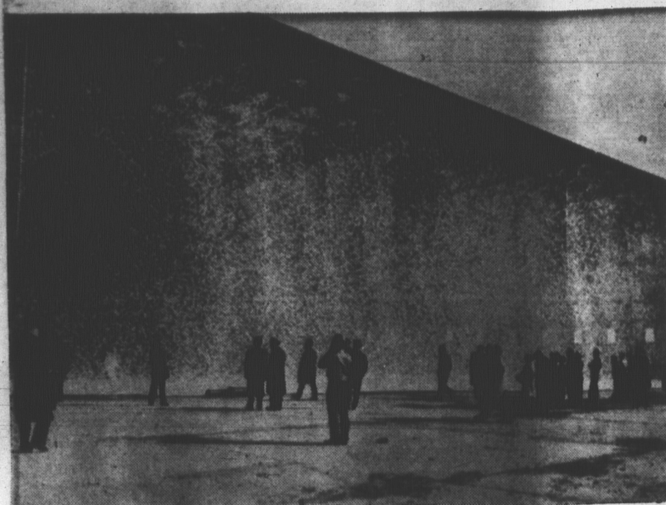
TESTING HANGER FOAM EXTINGUISHER SYSTEM
