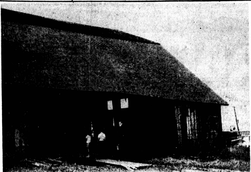
No, two elephants didn't just walk through the side of this building. This is a section of Summerside's Crystal Rink showing what is left of one wall and showing a section of about 35 feet which has been completely dismantled by vandals. This is the north side of the building which is adjacent to Court Street. As far as is known no police action has been taken. -Photo by Heckbert
