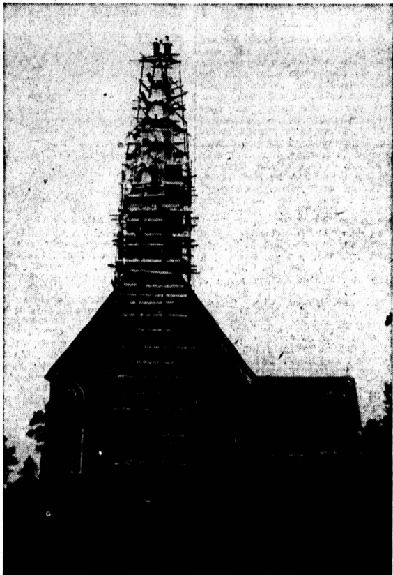
Shown above is a picture of the Sacred Heart Church at Alberton as it appeared recently while the steeple was being repainted. Mr. William Albert and Mr. Agurh McCabe can be seen on the staging 140 feet from the ground.
