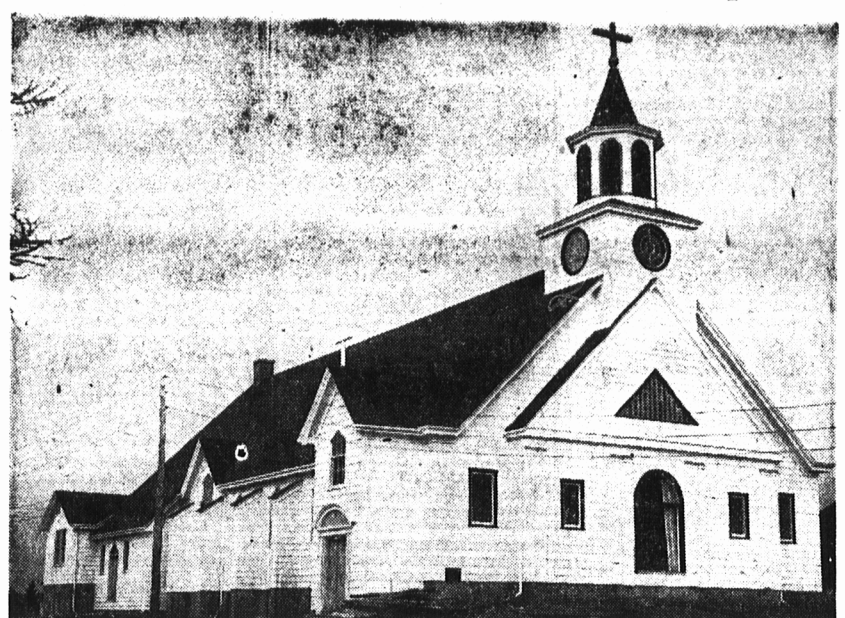
-Pictured above is the new Immaculate Conception Church at Wellington, now nearing completion. The new structure replaces the old church which was completely destroyed by fire on January 21st, 1951. Construction of the church began on June 21st of this year by M. F. Schurman Co. Ltd., Summerside, and it is expected that it will be ready for use about the middle of November. Most of the exterior work has been completed and the interior work will take considerable time to finish. When completed the new church will be one of the finest country churches in this Province. It will be heated by an air-conditioning unit and is 132 feet long and 46 feet in width. The spire reaches a height of 72 feet. Rev. Leonard MacDonald is the pastor of the parish.-(Photo by Wotton).
