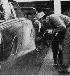
5. Enamelling. Now every joint, inside and out, is sealed by hand and the car is ready for enamelling. It gets not one but three complete coats and is thoroughly baked to produce a high-chip-resistant gloss.
