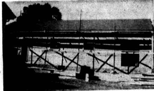
BUILD CHURCH HALL
