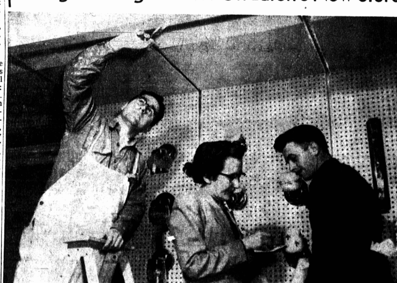
Putting the last finishing touches on the ceiling of lamp department of the new Eaton Store in Charlottetown is painter Dave Head. Mrs. A. Weatherbie and Lloyd Roundell go right on checking merchandise.
