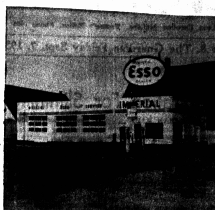
VIEW OF NEW STATION
