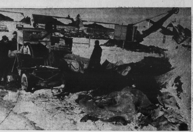
ARENA FOUNDATION BEING LAID AT ALBERTON
