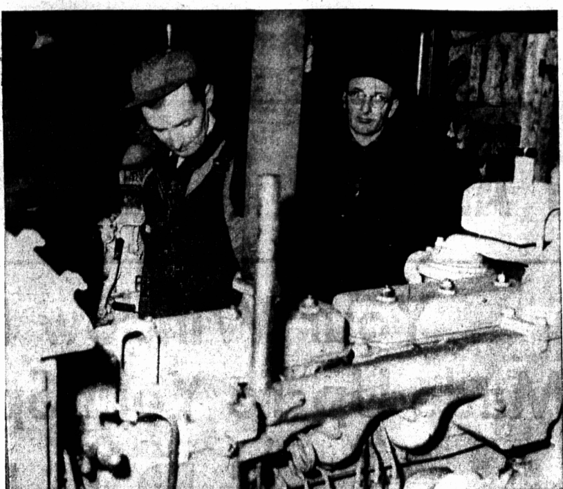
Adding To Alberton's Power Supply
