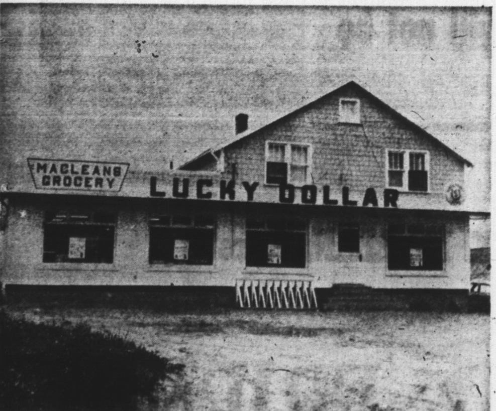
MacLean's new Lucky Dollar Store in Winsloe. The store with the sign of quality and value.
