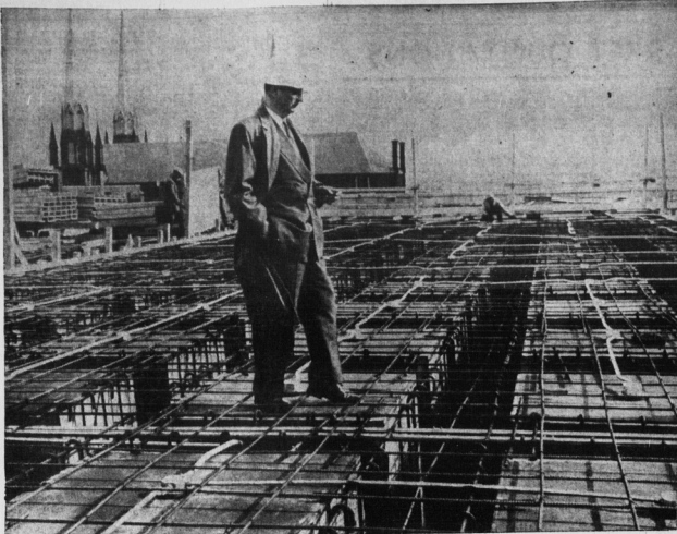
ROOF-POUR SCHEDULED TUESDAY
