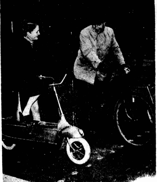
A Berlin husband who has more than a touch of "Sir Galahad" in his make-up conceived the idea for a new streamlined bicycle which would protect his wife from splashing. A refugee from the Soviet zone of Germany's eastern provinces, now under Czech control, Walter Fischer invented the bicycle which has a regular body with fenders to keep the driver's feet off dirt roads. It also has a small luggage compartment which will house a small power engine if so desired. Above, Mrs. Fischer is shown trying out her new sleek cycle in Berlin, while an admirer of new machine looks on.
