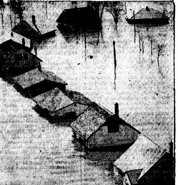
One of the dishearteningly common scenes in the Winnipeg flood area shows homes in the Willow Park section almost up to the eaves in water.
