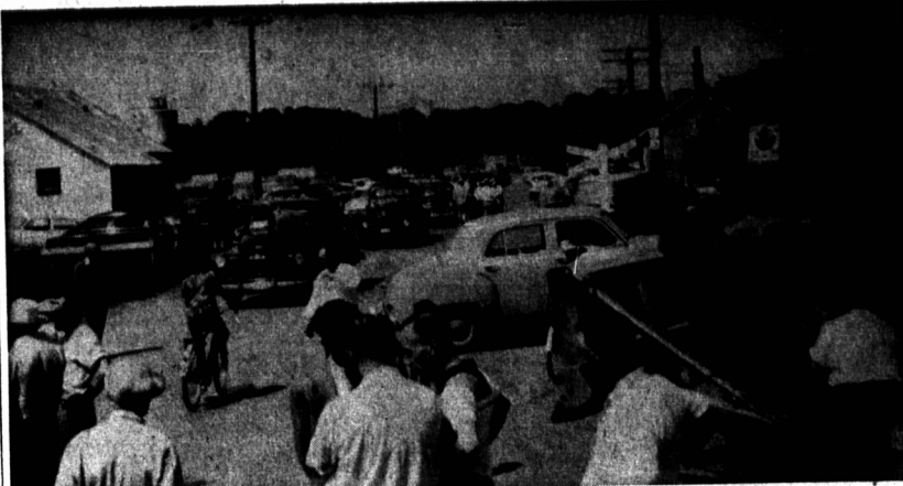
Traffic Piles Up While Bridge Closed
