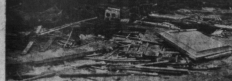
EXPLOSION SCENE IN ASBESTOS
