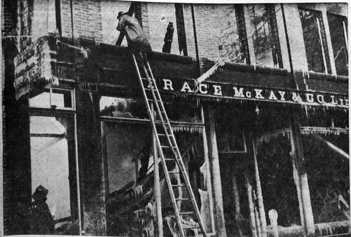
BUSINESS PREMISES COMPLETELY GUTTED BY FIRE
