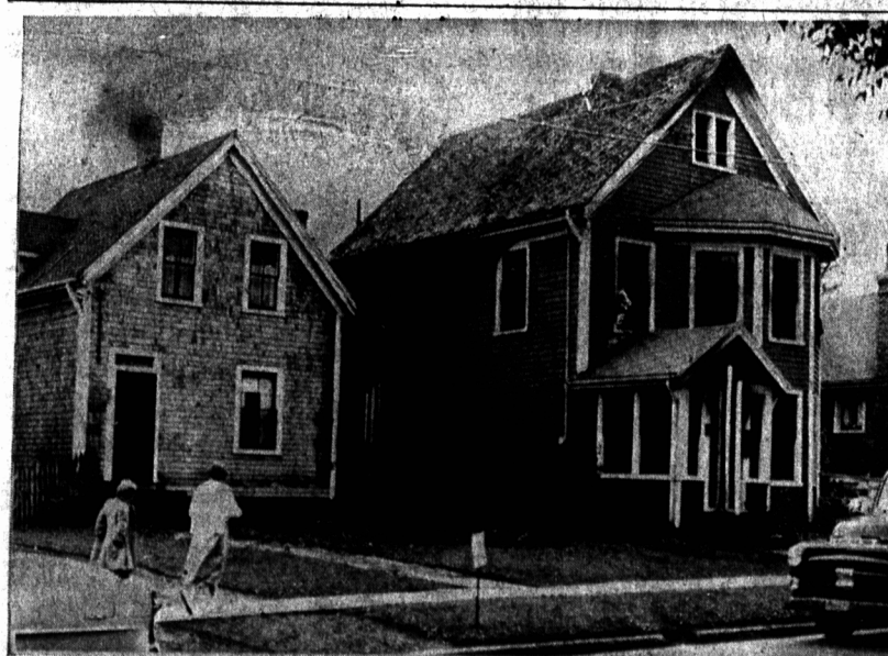
THIS FINE RESIDENCE on Fitzroy Street owned by Mrs. George Hennessy within minutes was completely gutted by a flash fire.
