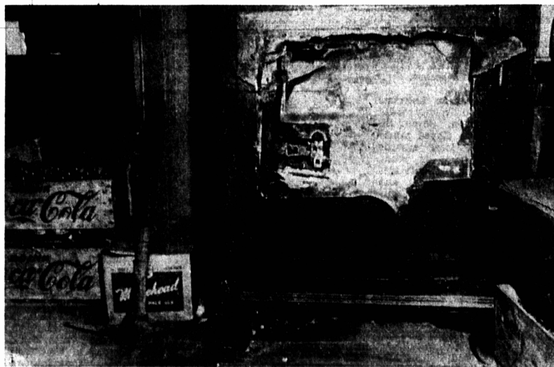
Above is the safe on which robbers worked at the dwelling-store of Mr. Lester H. Lavors of Georgetown Friday night and Saturday morning. They smashed a hole about five inches square in the upper left corner. Other damage was caused later by police opening the safe to see what had been taken after the robbers wrecked the lock, making it impossible to open. The robbers escaped with some $625 from all sources. Photo by Pepler, Montague.
