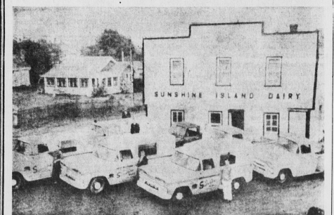
Sunshine Island Dairy Modern Plant
