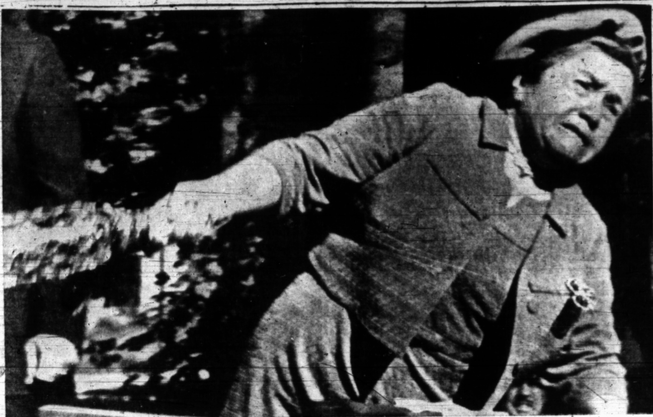
CHARLOTTE GIVES SEWER SMASHING START
