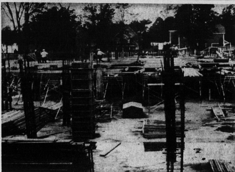
PROVINCIAL GOVERNMENT OFFICE BUILDING UNDERWAY
