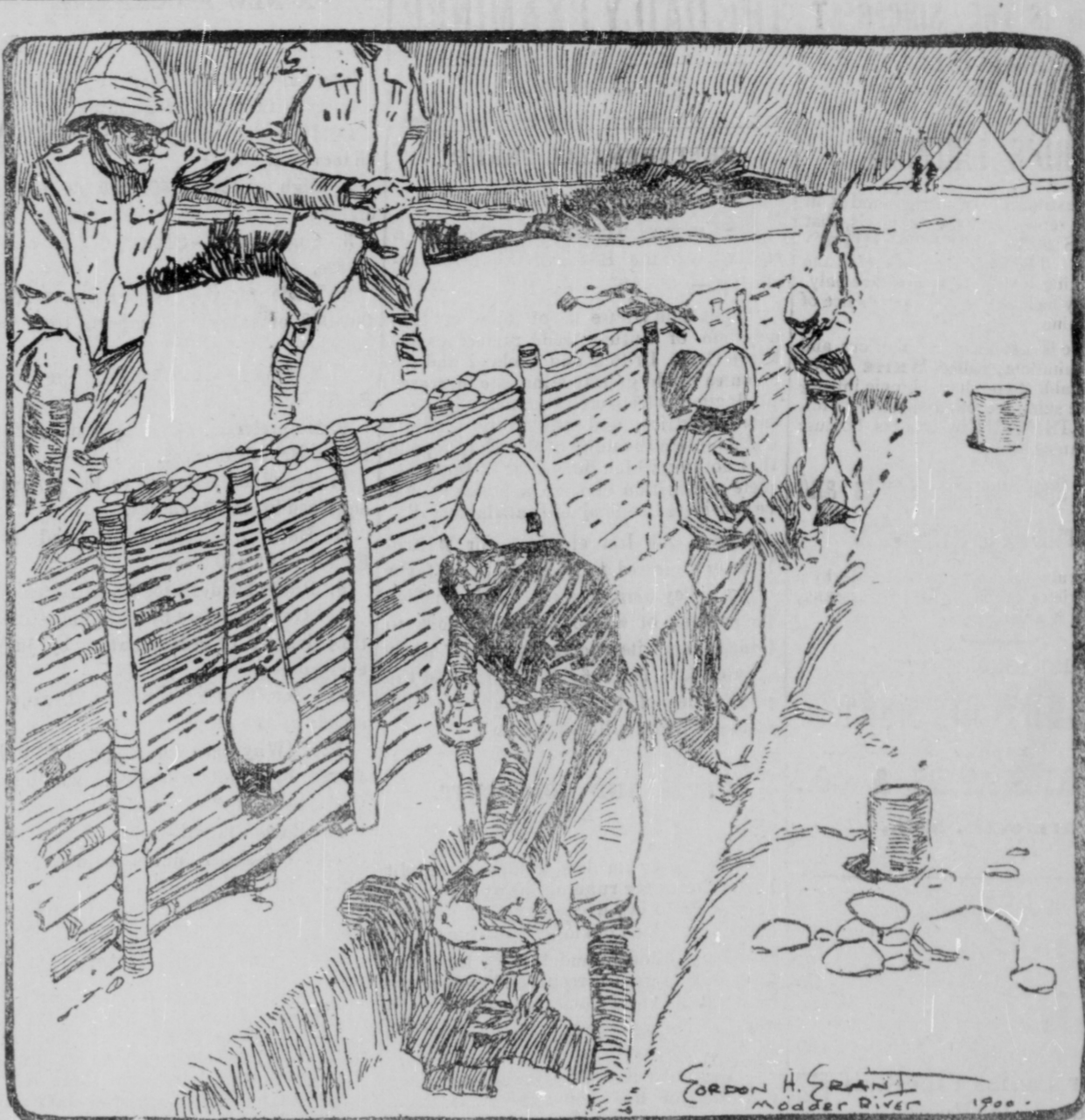
PUTTING THE MODDER IN DEFENSIVE ORDER AGAINST BOER REAR ATTACKS. In his campaign of advance Lord Roberts has also been especially careful to protect his line of communication in pursuance of that plan the Modder river, which flows around the north and east of Bloemfontien, has been strongly fortified. The brush to the left of the picture marks the river bank along which breastworks are being put up to protect the garrison that shall be left after the column has advanced.—Boston Globe.
