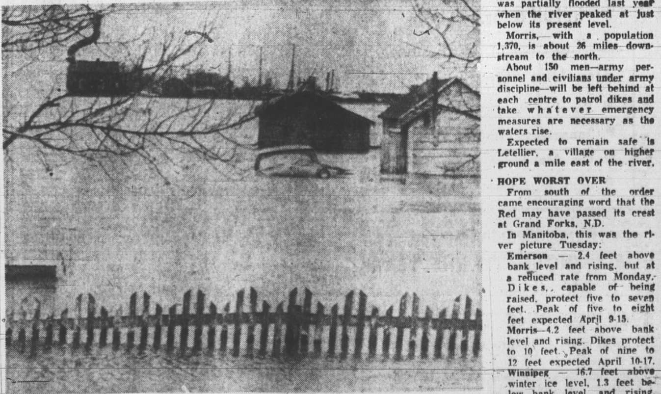
FLOODING BECAME more than a threat at Morris, Man., Tuesday as the Red River spilled over its banks, half-submerging buildings and cars.
