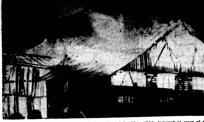
Four hundred turkeys were burned to death in blaze which destroyed 14 years of work. $32,000 fire which gutted barn on farm of Irwin to develop a new breed of birds. Flames from fire, from at Hespeler, Ont. Defective wiring was seen above, could be seen 20 miles away.
