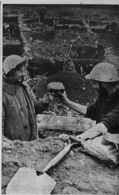
RESTORATION UNDERWAY AT LOUISBURG
