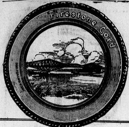
One of the world's longest bridges—nearly two thirds of a mile—spanning the St. Lawrence at Quebec.
