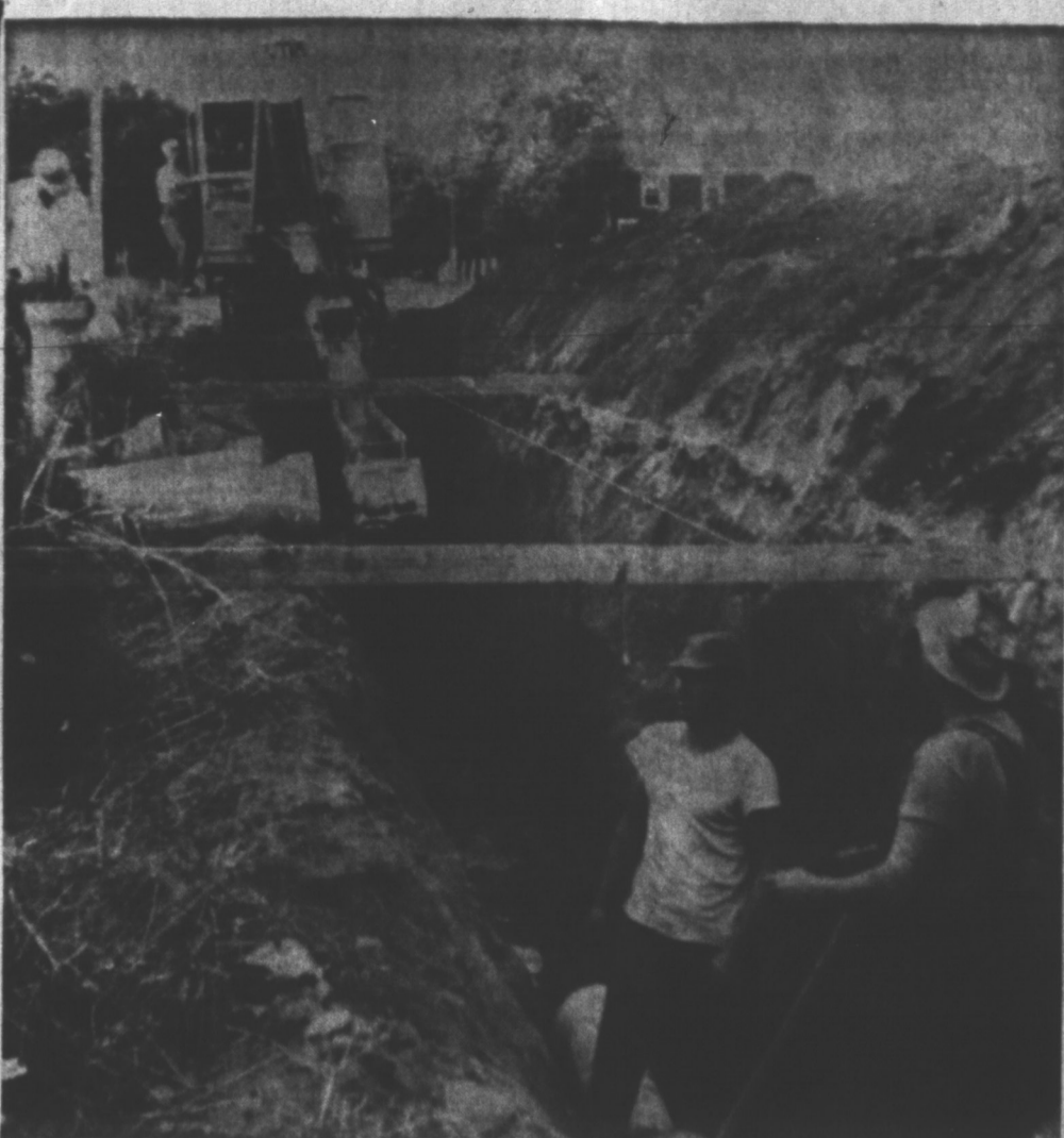
MASSIVE SEWERAGE INSTALLATION WAS STARTED IN TIGNISH IN '61
