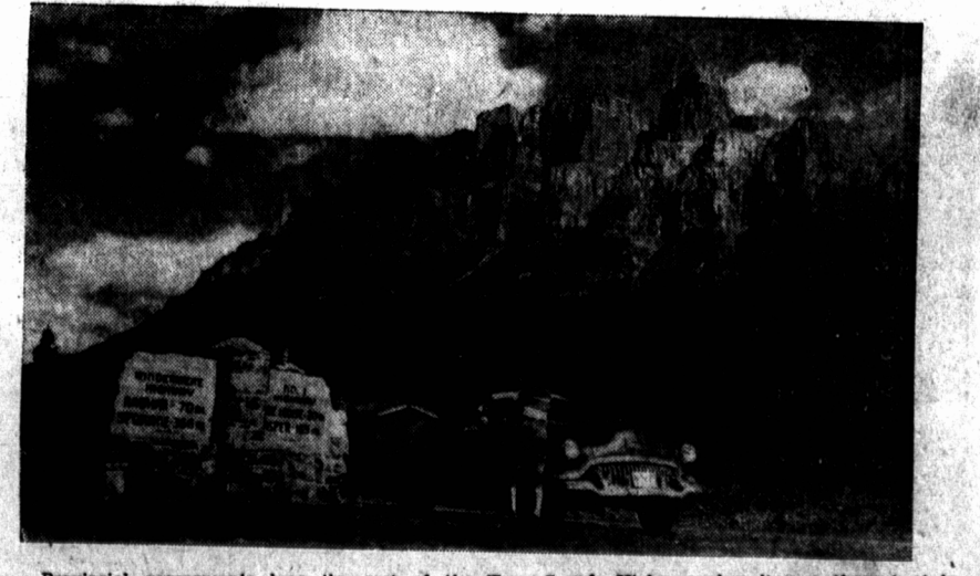
Provincial governments bear the cost of the Trans-Canada Highway when it goes through their provinces. But the federal government alone has responsibility for building and maintenance of the 83 miles of highway through the scenic Banff and Yoho National Parks in the Canadian Rockies. The mountain in the picture is Mount Eisenhower, named after President Ike when he was a general.
