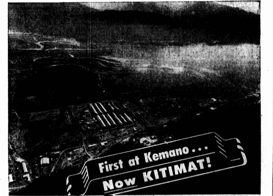
Aerial view of first stages of aluminum smelter now nearing completion at Kitimat, B.C.
