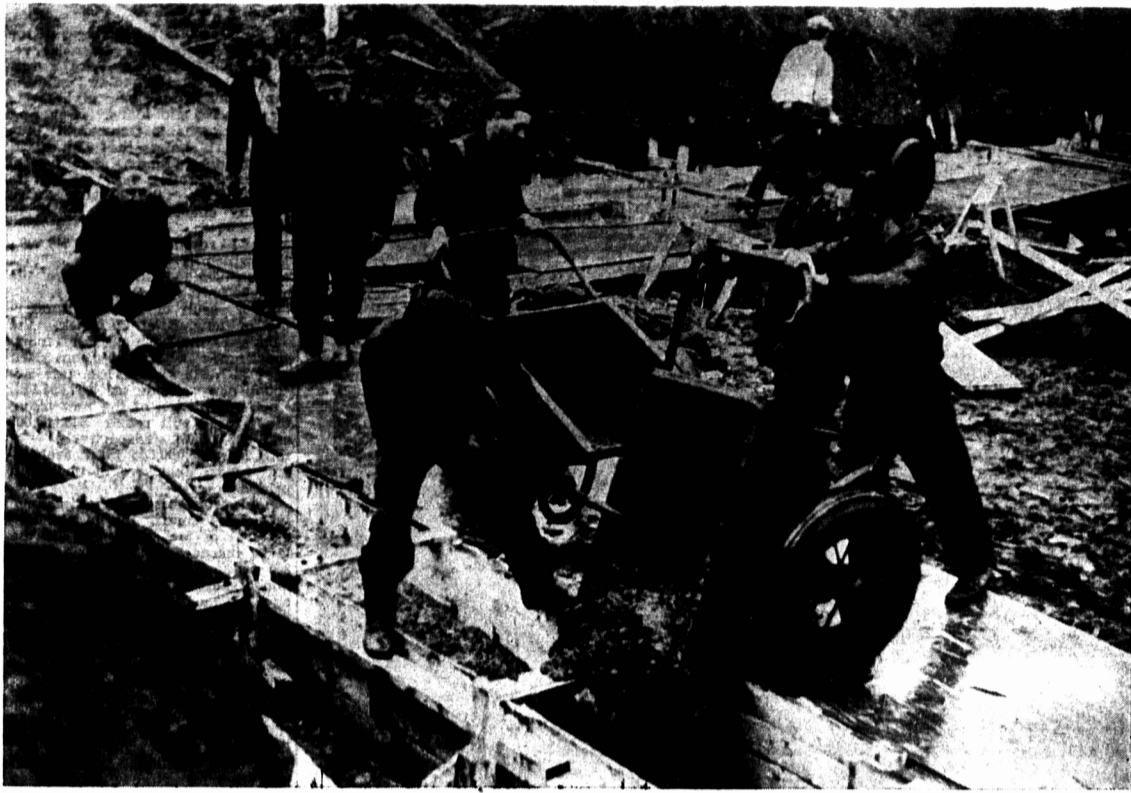
Gus Savoy, Superintendent of Construction for Anglin Norcross (Maritime) Limited (left) with Foremen Beaudry and Phelan check the first buggy runs on Saturday morning.
