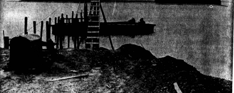
NEW WEST RIVER BRIDGE UNDER CONSTRUCTION
