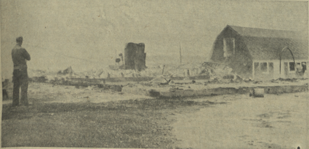
FIRE LEVELS HOME A fire of undetermined origin raged through the home of Mr. and Mrs. Frank Kohout of North Tryon, Tuesday morning and left nothing but a stark chimney standing amid the ruins. A bucket brigade and a mechanical potato sparer, converted for the moment to a fire hose, saved the barn in the rear.
