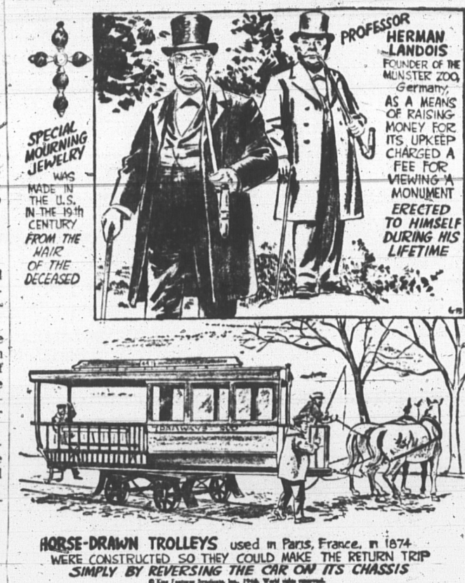
HORSE-DRAWN TROLLEYS used in Paris, France, in 1874. WERE CONSTRUCTED SO THEY COULD MAKE THE RETURN TRIP SIMPLY BY REVERSING THE CAR ON ITS CHASSIS.
