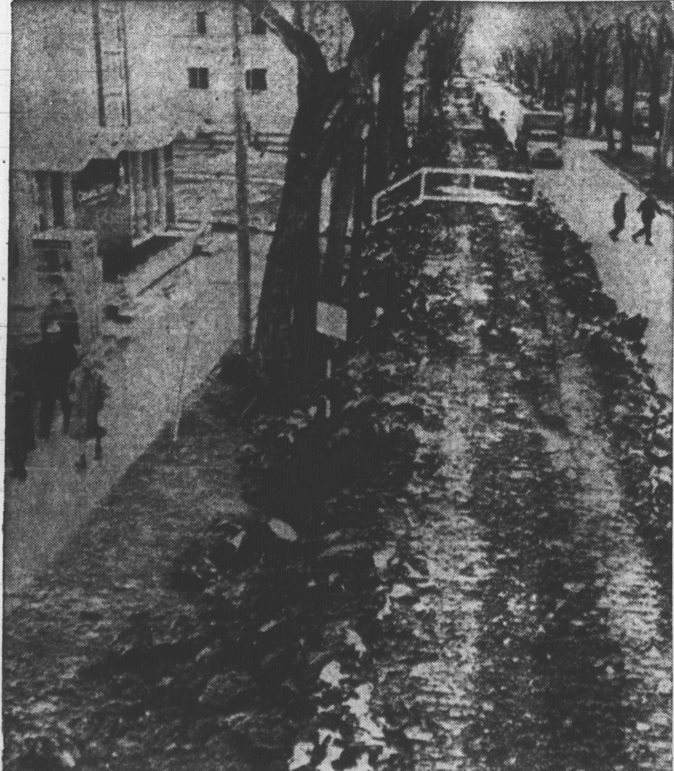
EARTH DIKE IS READY FOR FLOOD
