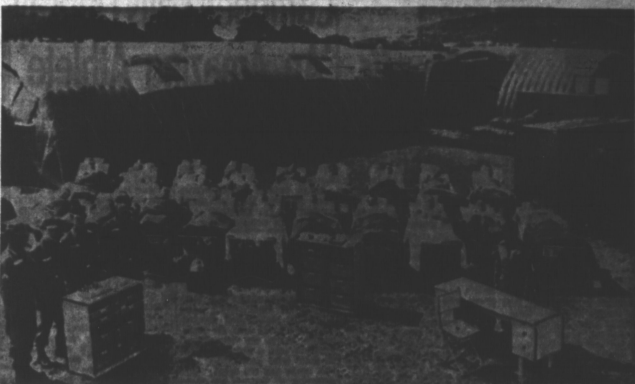
ARMY HOSPITAL, would be patients, nurses and orderlies take to the sun as they show just how much is packed in a box. This new hospital in a box was shown Wednesday by the Brooke Army Hospital at Antonio, Texas. This inflated hospital, background, and all the beds, tables, desk, chair and other equipment goes into the box at right. This mobile field hospital can be set up in 30 minutes. Thursday the U.S. Army was host to the House of Representatives, armed services committee and representatives of industry and medicine to show off this new hospital concept that the army wants for its strike units and thinks is a prime development for civil defence. (AP Wirephoto)
