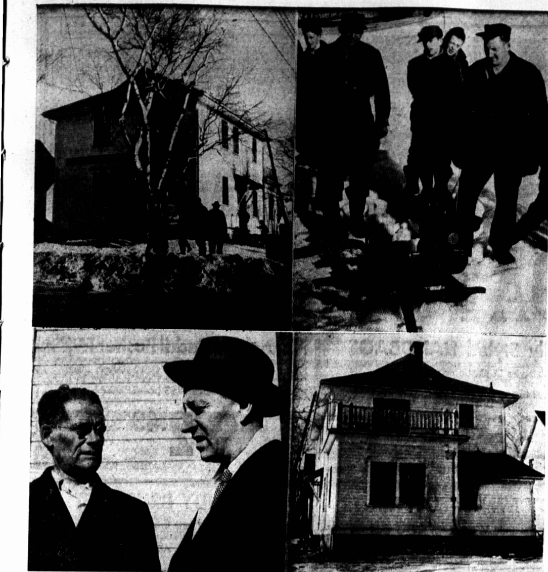
TOP LEFT - The front and side of the Bank of Nova Scotia building in the centre of Victoria village where a fire caused extensive damage yesterday morning. TOP RIGHT - Ralph Myers and Elmer Macdonald, two members of the Crapaud volunteer fire department, are seen operating one of the department's portable engines which were instrumental in preventing the complete destruction of the Bank of Nova Scotia building at Victoria. LOWER LEFT - Transferred to Bath, N.B., as bank manager, and scheduled to leave for there next Tuesday, Donald Hart, face smudged with smoke and soot after he and his family escaped yesterday from their burning home, discusses the effects of the fire at Victoria with Ralph De Grasse, who is scheduled to replace Mr. Hart as manager of the Crapaud and Victoria banks next week. LOWER RIGHT - Back of the bank building at Victoria shows black and broken windows where fire raged until brought under control. Balcony above is spot from where Mrs. Hart and her six-year-old daughter were rescued. Photo by Wotton
