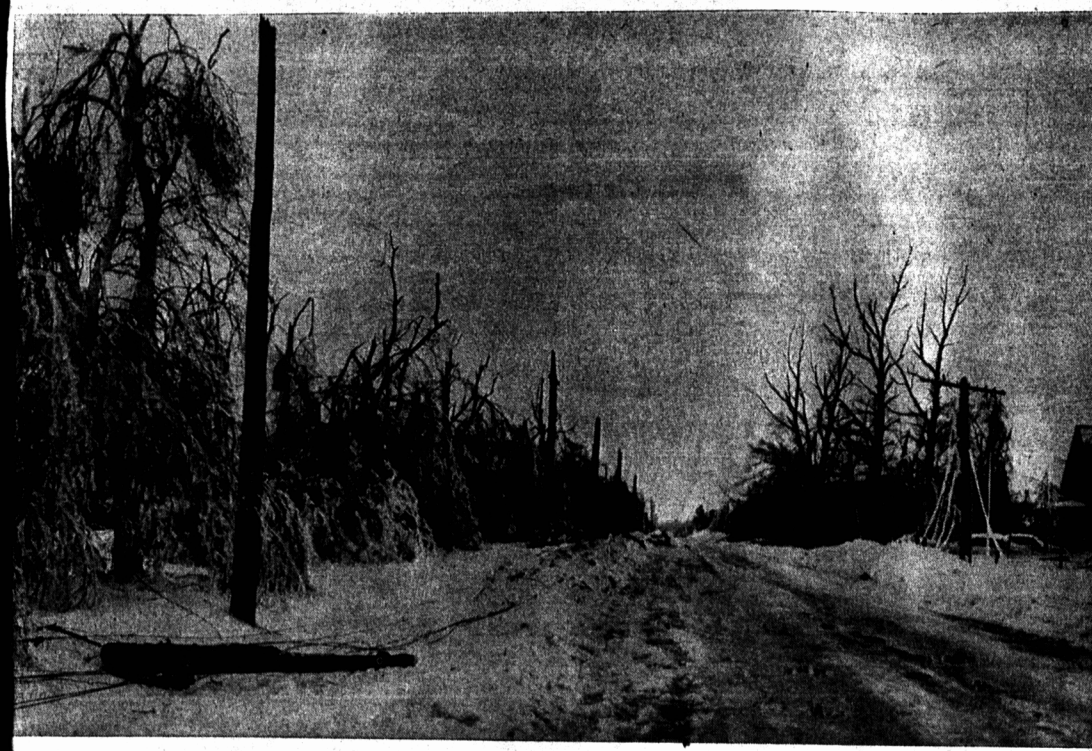
ALBERTON STREET AFTER THE ICE DID ITS WORK This street at Alberton, near the Princess Pat Theatre shows power poles with the tops broken off and all wires and transformers on the ground. Most telephone wires across the street are also down and the ornamental trees are broken wrecks.
