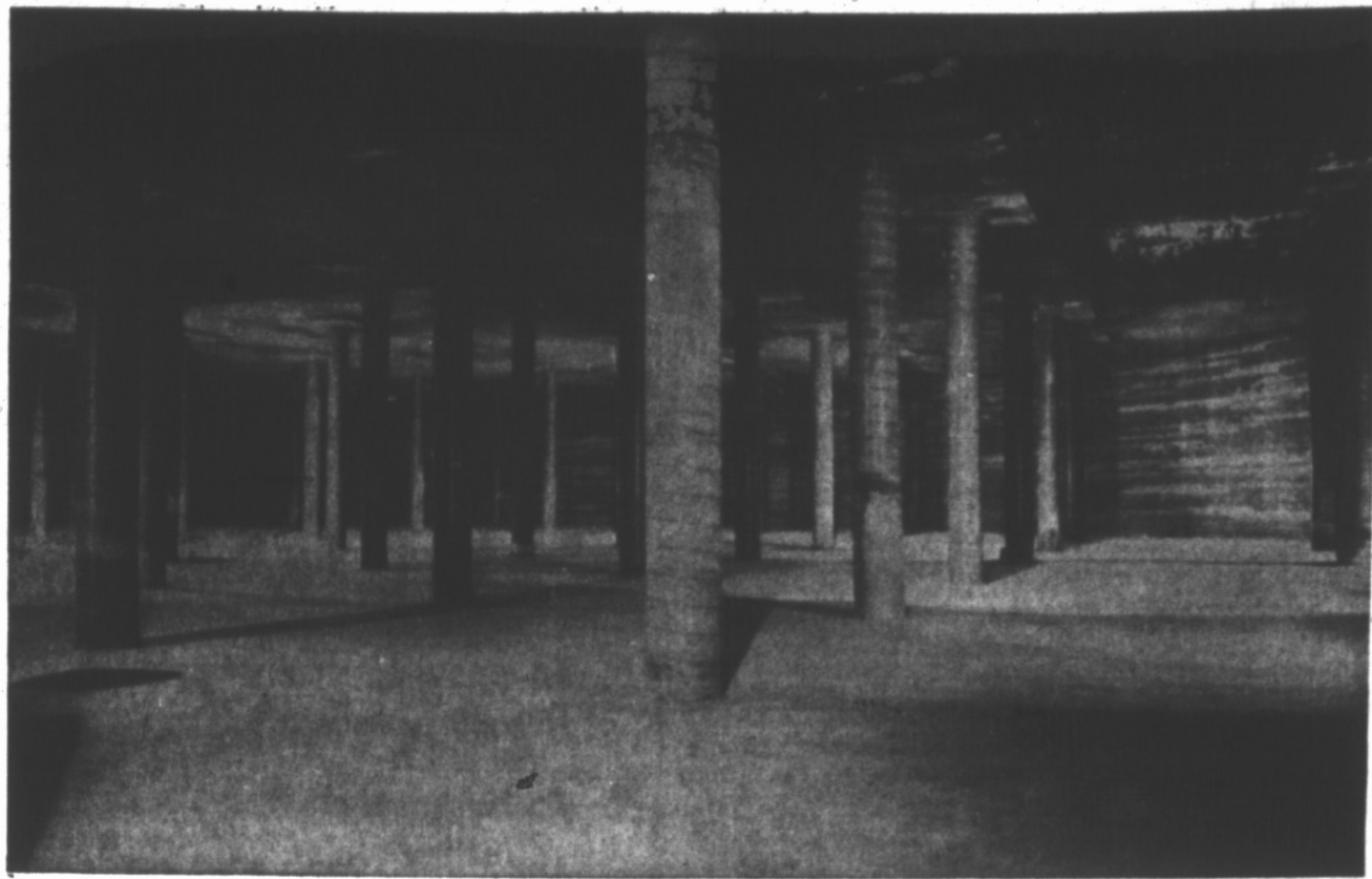
INTERIOR CITY'S NEW WATER RESERVOIR
