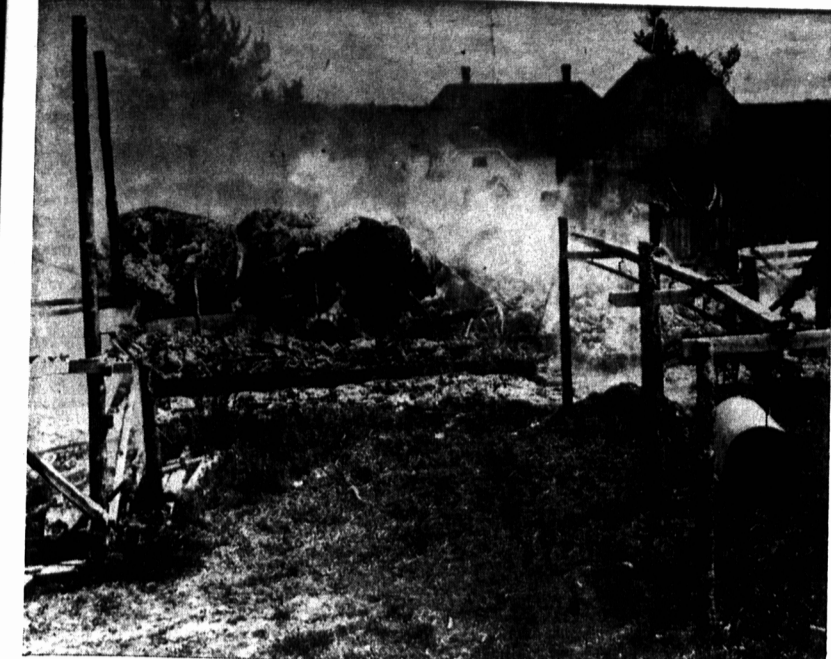
WHAT REMAINS of the barn on fire, is a heap of smoldering hay, twisted metal where the cow stall were located and a few smoking corner posts.
