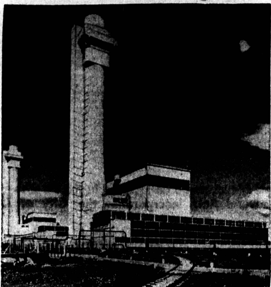
First photos released by Britain of its atom factories include this view of Windscale plutonium producing plant, staffed by nearly 5,000 men, including 300 architects and engineers. The filters at the top of the 400-foot chimneys prevent the escape of the last traces of radioactive matter.
