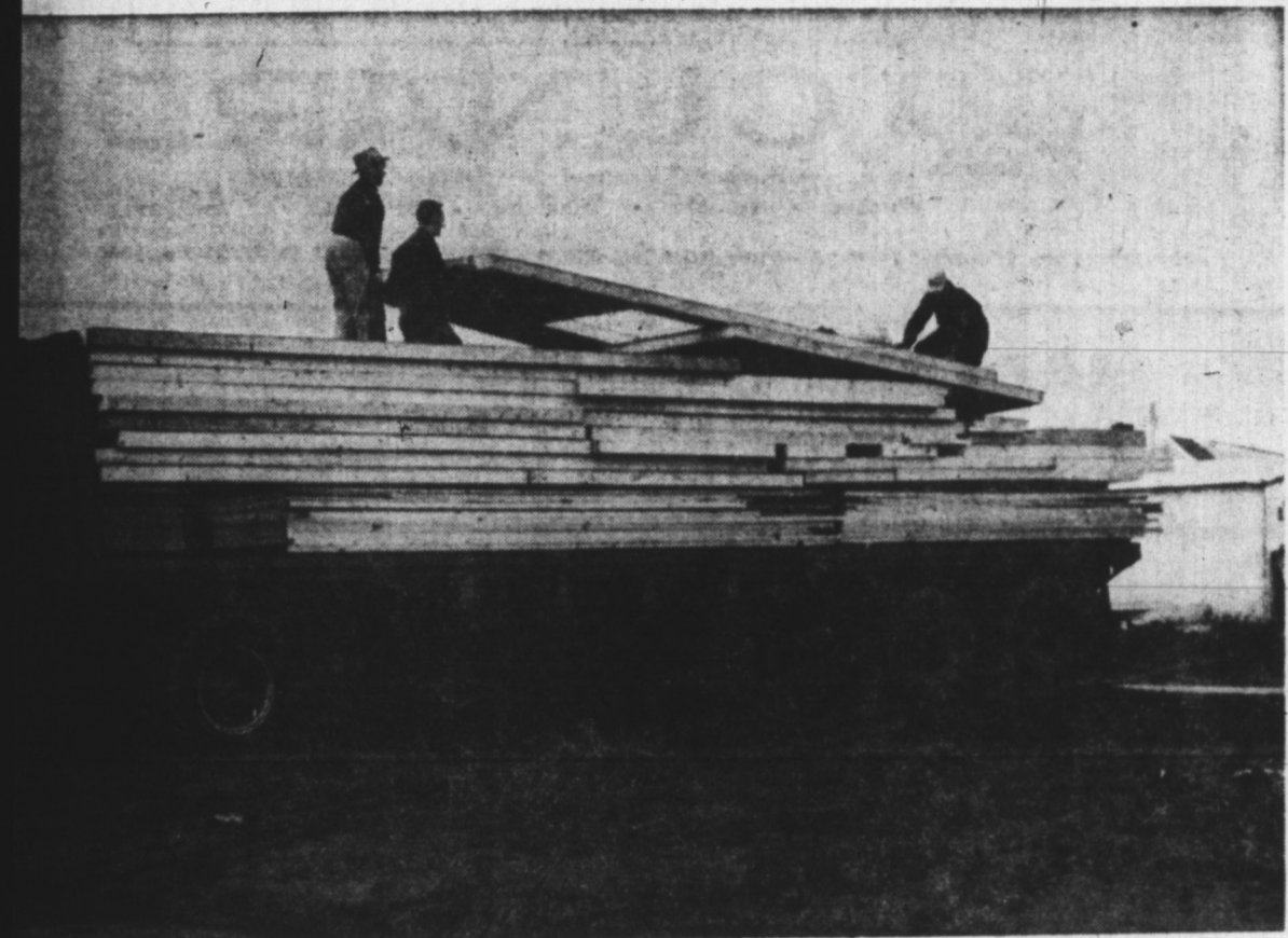
7:15 a.m. The truck arrives at the job site loaded with the component parts for the house. This photo was taken at 7:15 a.m. and shows the first section being unloaded.
