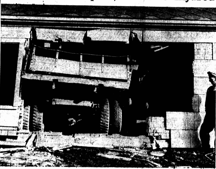
Finally stopped by several tons of canned vegetables, only the back end of a three-ton gravel truck is seen after it smashed through the side of the canning plant of Campbell & Burns at Central Bedouque yesterday afternoon. No one was injured. The accident occurred when the truck driven by John Anderson of Breadalbane left the pavement and continued on for some distance through the side of the building and ended up amid 1,000 cases of canned vegetables to which considerable damage was caused. See story and other pictures on page 13. (Photo by Wotton).
