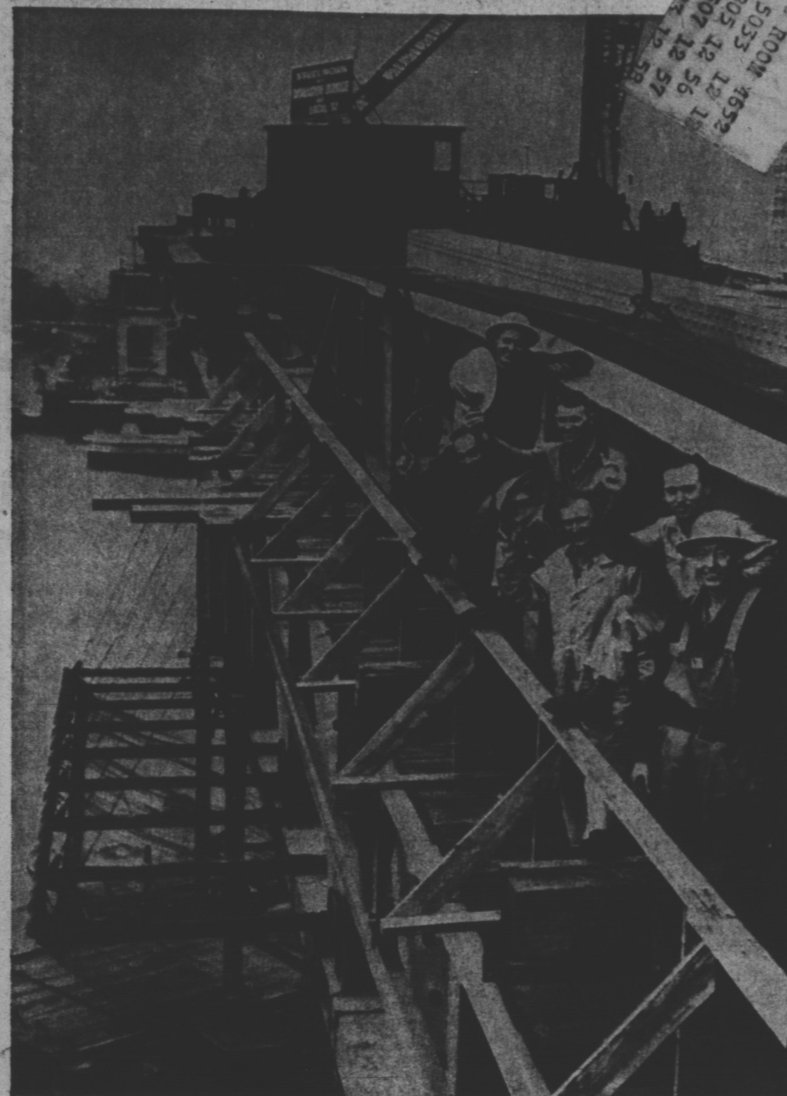
BRIDGE IS BEING REBUILT
