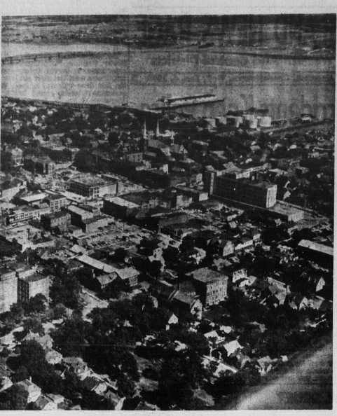
AERIAL VIEW, CHARLOTTETOWN
