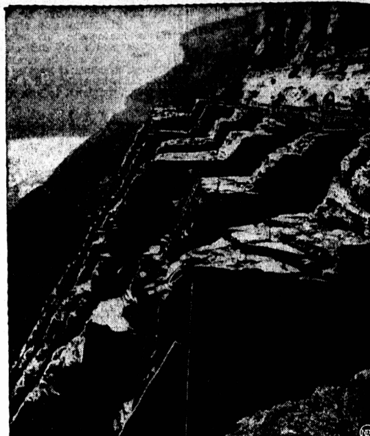
POWER PENSTOCKS: This is part of the rock-blasting being done on the shore of the Niagara River (seen faintly at left) for the seven penstocks that will bring water from Niagara Falls to a new generating station to create 700,000 horsepower.
