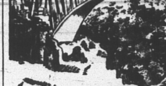
PAUL SAUER BRIDGE over the St. Lawrence River, South West, which spans a CHAIN 400 FEET IS SUPPORTED BY 2 HIVE CROSSES WHICH WERE SUNK VERTICALLY INTO THE ROCK—AND THEN BENT INTO AN ARCH—JOINING PERFECTLY AT THE CENTER
